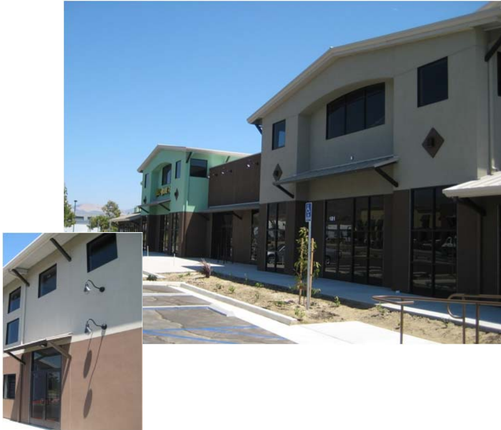
Tank Farm Design Center San Luis Obispo, California
